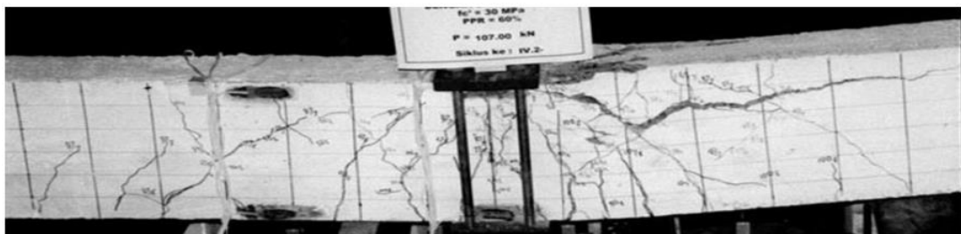
Figure 2.29: Crack pattern of original specimens (Budiono et al., 2000)
