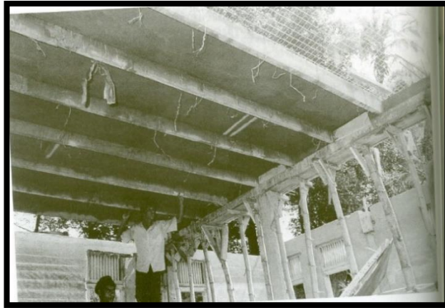
Figure 2.1: First slab construction at the NERD center
