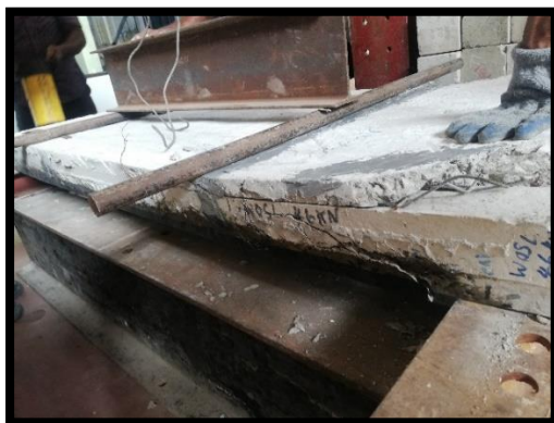
Figure 5.8: Models failed by de-bonding of CFRP
