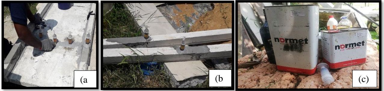
Figure 4.7: Inject epoxy resin (a) for composite panels (b) for pre-stressed beams (c) low viscosity long pot life epoxy injection resin, TamRez 220 TG
