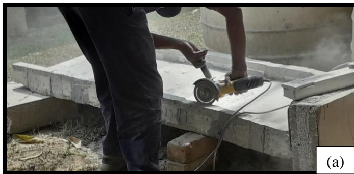
Figure 4.9: Surface preparation (a) Grinding off weak layer of concrete (b) Appearance of ground concrete surface.
