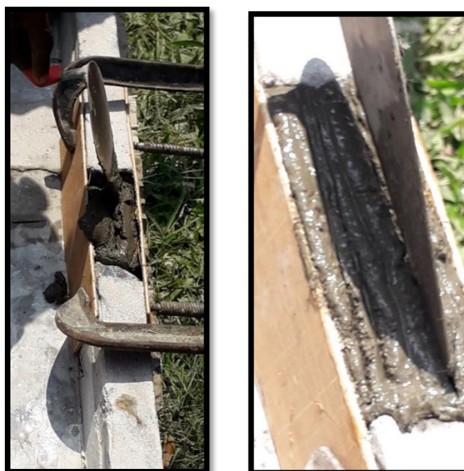
Figure 4.6: Repairing of cracks using structural repair mortar
