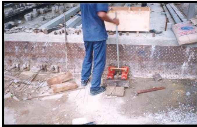
Figure 2.5: Stressing wires using special jacking arrangement.
