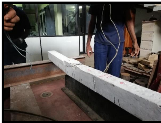
Figure 5.3: Cracking on pre-stressed beams
