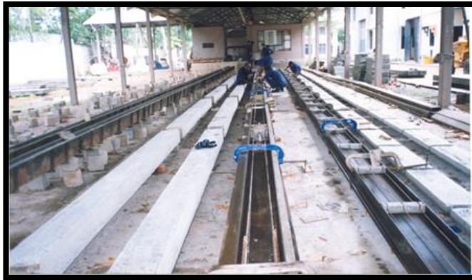
Figure 2.6: Longline method of casting
