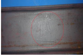
Figure 3: Crack propagation zone under loading □
