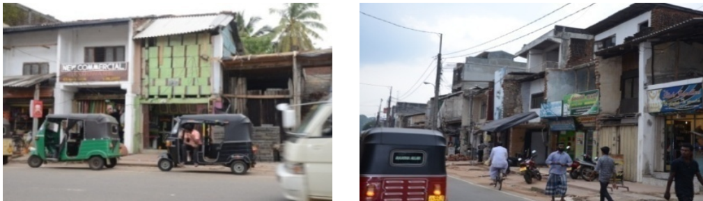
Figure 6: Chaotic built forms abandoned buildings and deteriorated urban fabric – City of Matale Source- author
