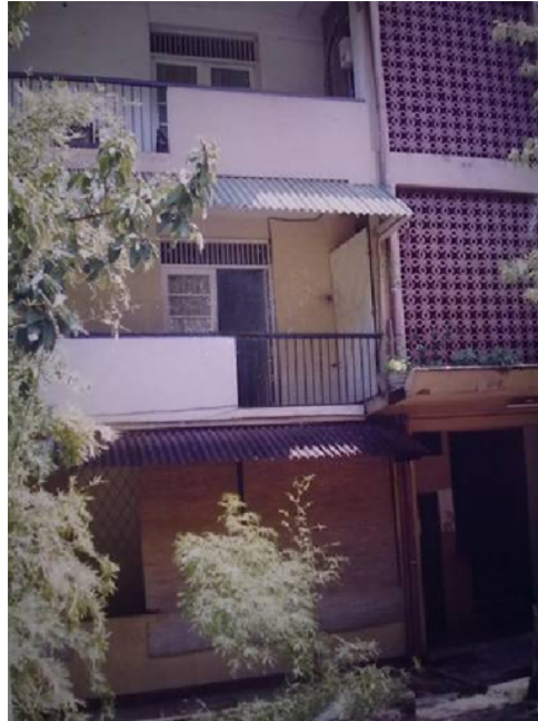
Fig. 6: Elvitigala Housing scheme. The stair case that serves two adjacent residential stacks and its landings are located behind the red cement grill which ensures visual connectivity with the semi-private green space below.
