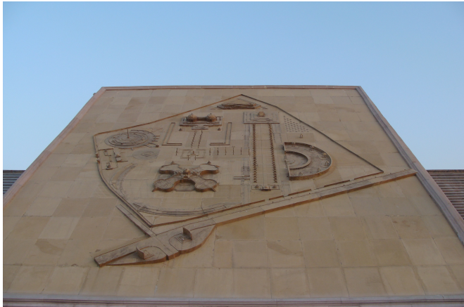
Fig. No. 11 The Ambedkar Samajik Parivartan Sthal model at the termination of the elephant flanked axis. Architecture becomes the end itself!!! Source: Author
