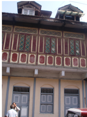
Fig.26: Str. on D M Road Source: The Author
