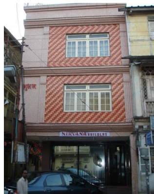
Fig. 33: Incongruent renovation Source: The Author
