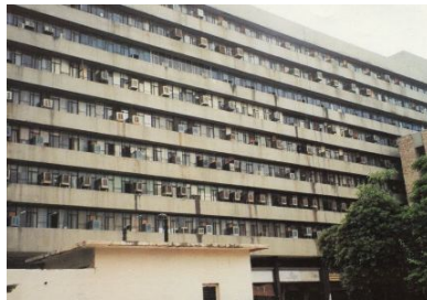
Fig. 6: A typical office building Source: The Author
