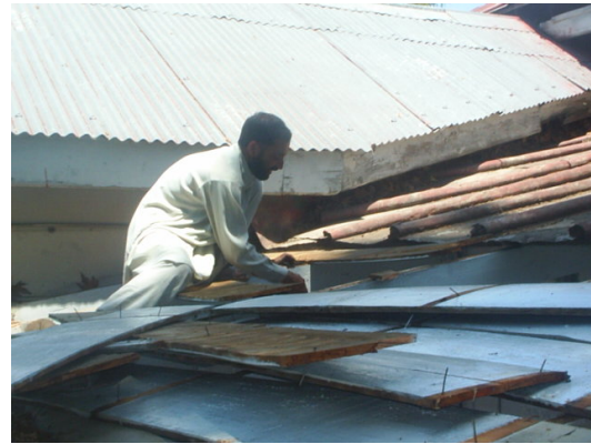
Fig. 5: Commissioner House Roof Inside Source: Author
