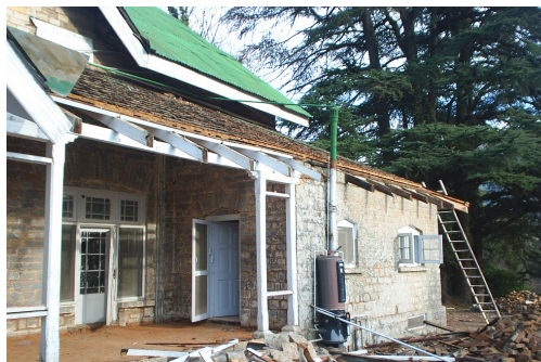
Fig. 4: Frontier House Back Side View Source: Author
