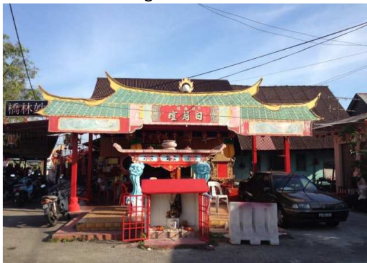
Fig. 3: Lim Jetty Temple Source: Author
