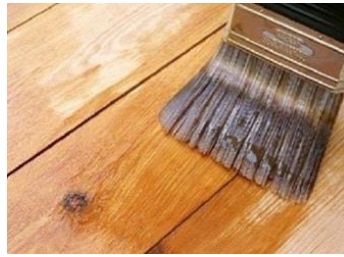
Figure 15:Brushing treatment
