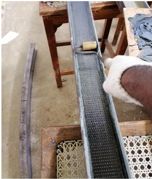
Figure 6.4. Pressing of CFRP using a roller
