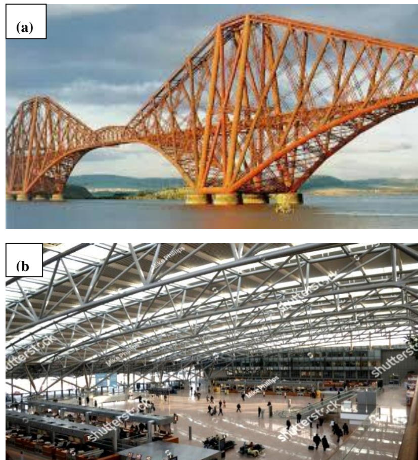
Figure 4.1. Structures constructed using SCHS curved in elevation (a) Firth of Forth bridge (b) Hamburg airport roof
