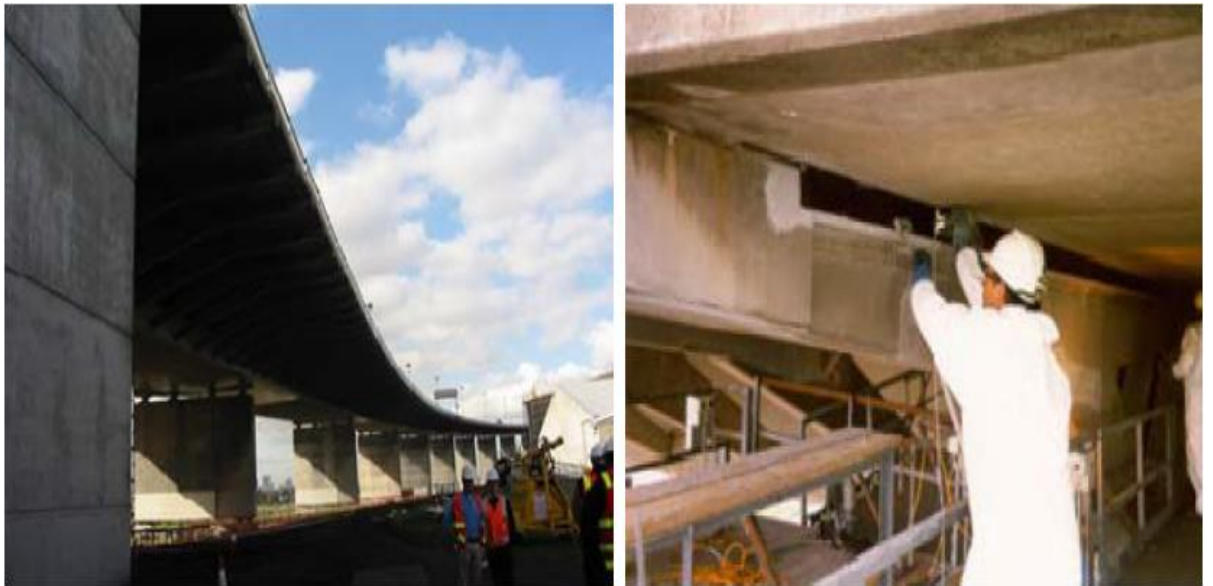
Figure 2.31. CFRP strengthening of West Gate bridge, Melbourne, Australia (Gamage 2009)
