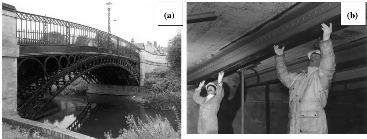
Figure 2.29. (a) Tickford bridge, Buckinghamshire, UK; (b) Installation of CFRP plates at Slattocks canal bridge, UK (L C Hollaway and J Cadei 2002).
