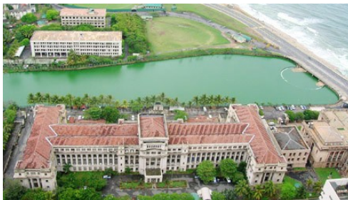
Fig 20: east beira canal-penetration A [source-SumuduGajanayake]
