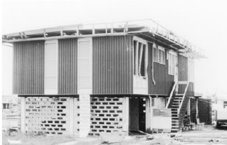
Figure 2.11 - Survived metal cladding of a house ( Walker, 1975 )
