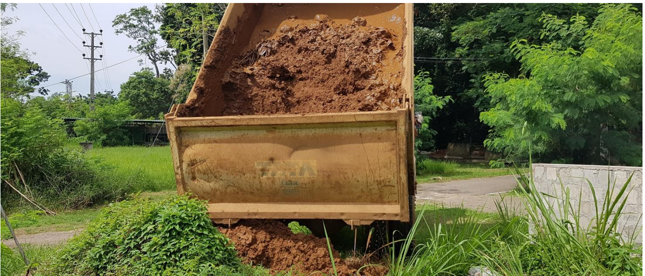
Figure 2.4; Removal of Water Treatment Sludge to Dumping Yards
