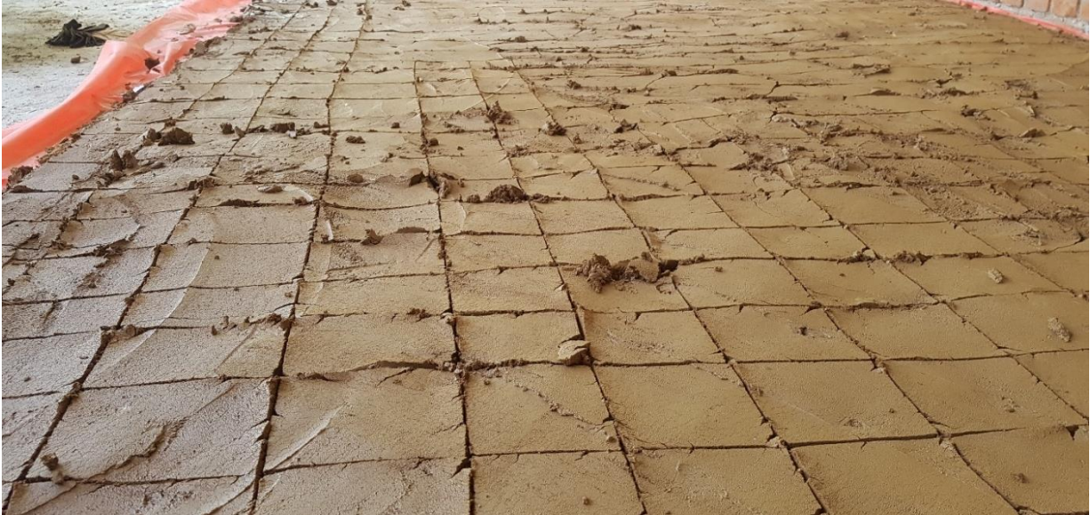
Figure 3.11; Wet sludge laid on floor and cut to 75 x 75mm
