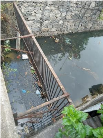
Figure 4.7: Water channel opening through a trash rack close to NFH
