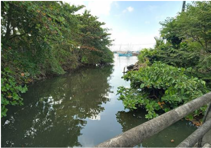
Figure 4.8: Water channel directly opening into the BFH
