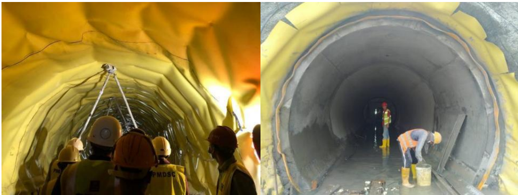
Figure 5: Applying of tunnel waterproofing
