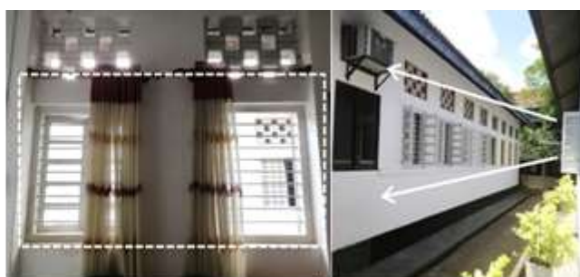
Figure 7, Existing Window and the immediate front of the Staff Room
