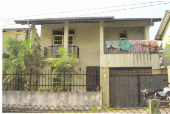
Plate 64- Front view of the house
