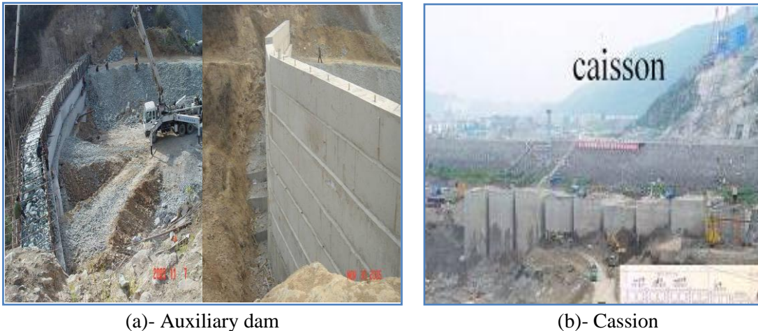
Figure 5 : Caisson backfill and Auxiliary dam examples
