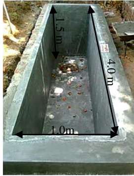
Figure 1: Constructed Lysimeter at Meewathura research site
