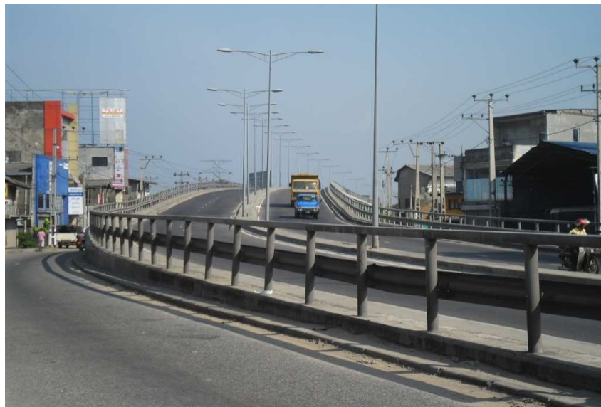
Figure 4 The completed expressway without expansion joints
