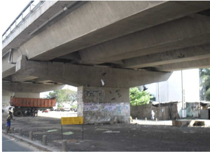
Figure 6 The completed bridge with 5.5 m cantilevers supporting the wider roadway
