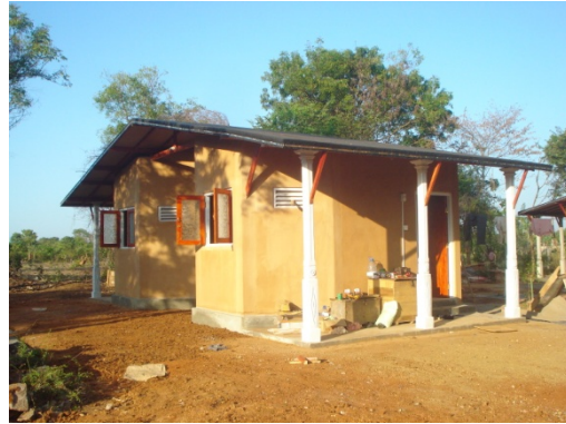
Figure 1: The completed house
