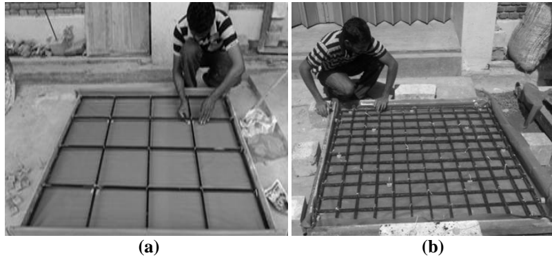
Figure 3: Palmyrah Reinforcement Nets of Slab 1 (a) and Slab 2 (b)
