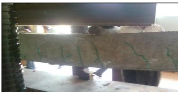
Figure 17: Flexural cracks in control beam
