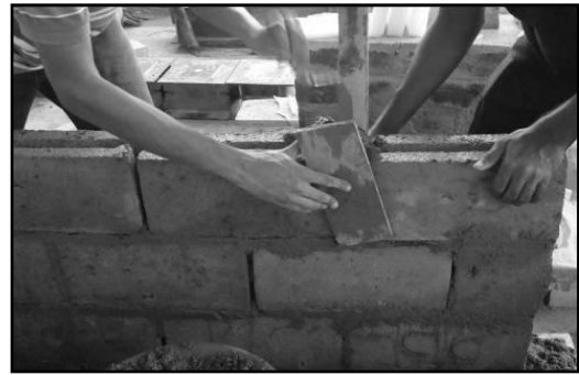
Figure 3– Casting the masonry wall panel
