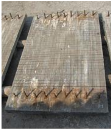
(a) Top (blast-receiving) face
