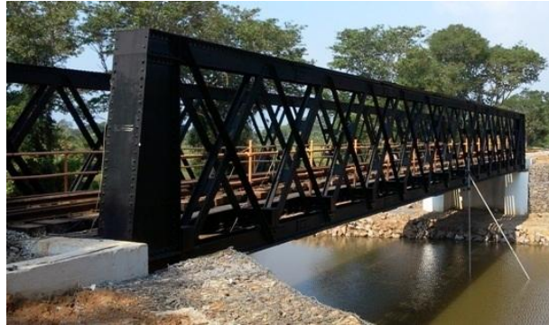
Figure 1 – Railway Bridge No. 2, Puttalam after repair & retrofitting.
