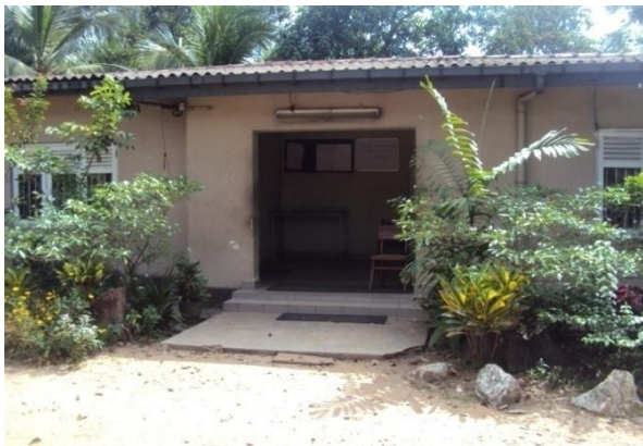
Figure 8 - Selected brick work building (Veterinary Office at Gampaha)
