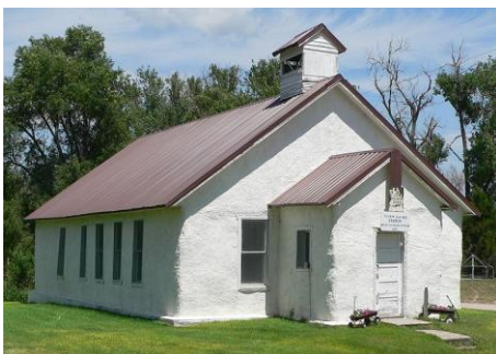
Figure 1 - Old straw bale Pilgrim Holiness Church in Arthur, Nebraska constructed in 1928
