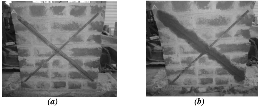
Figure 3: Installation of steel bracings on the wall surface
