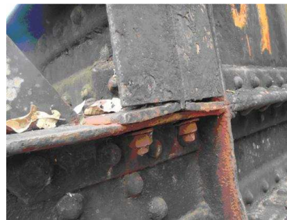
Defective connections
