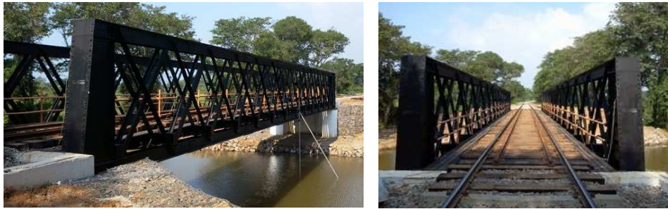
Figure 4 Bridge after improvement works
