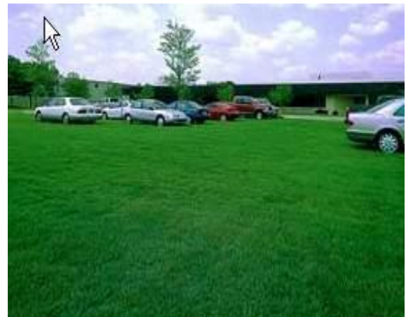
Figure 7: Pervious concrete car park, plated grasse on top of concrete.
