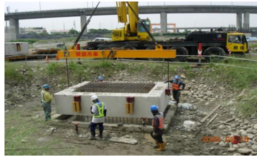
Fig.12 Precast pier erection
