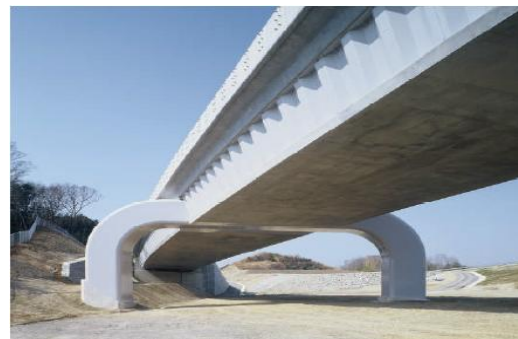
Fig.10 Bridge with corrugated web
