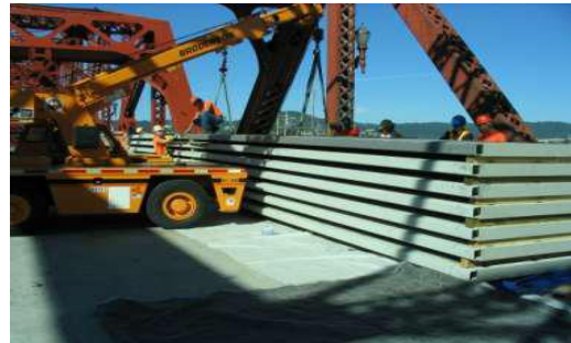
Fig.6 FRP deck erection
