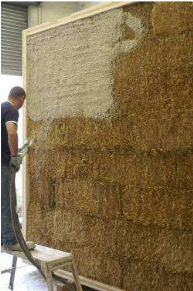
Figure 3. Spraying lime render on ModCell panel
