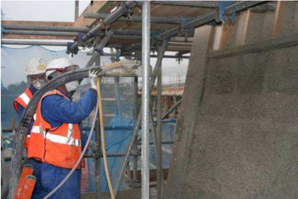
Figure 2. Spraying hemp-lime (Lime Technology Ltd)
