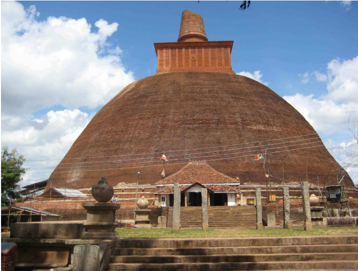
Fig. 7. Jetavana Stupa (3 rd century AD) After Conservation
