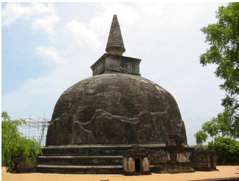
Fig. 8. Kiriwehera (12 th century AD) Showing Original Plaster
