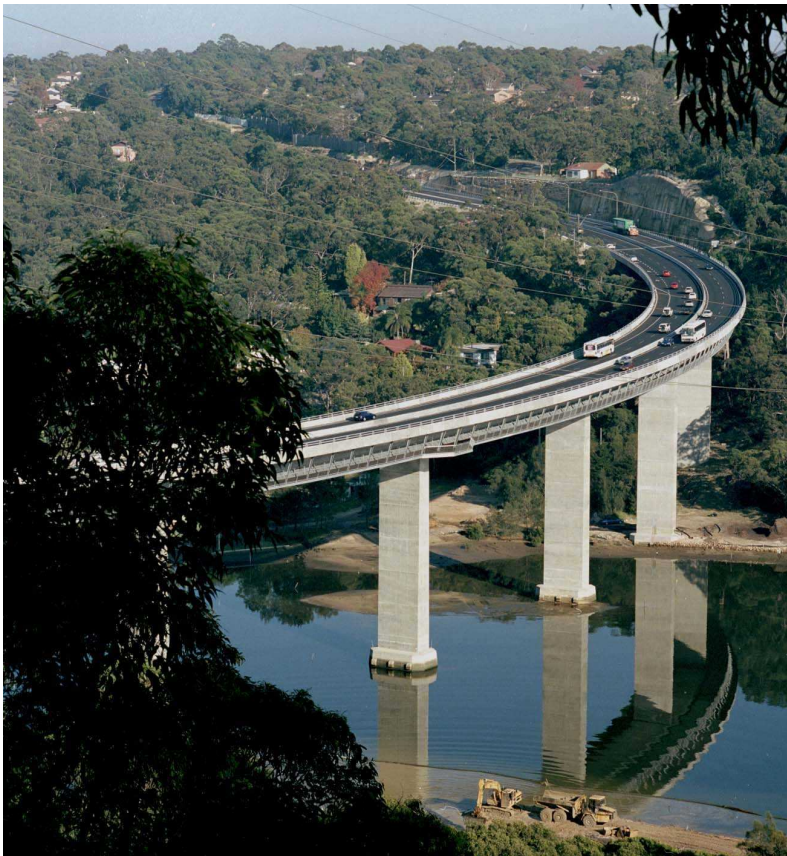
Woronora River Bridge
