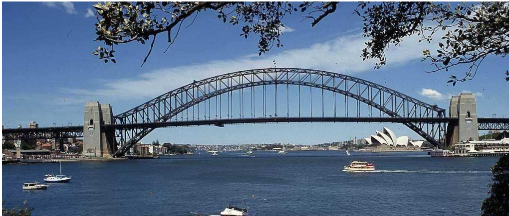
The Harbour Bridge
