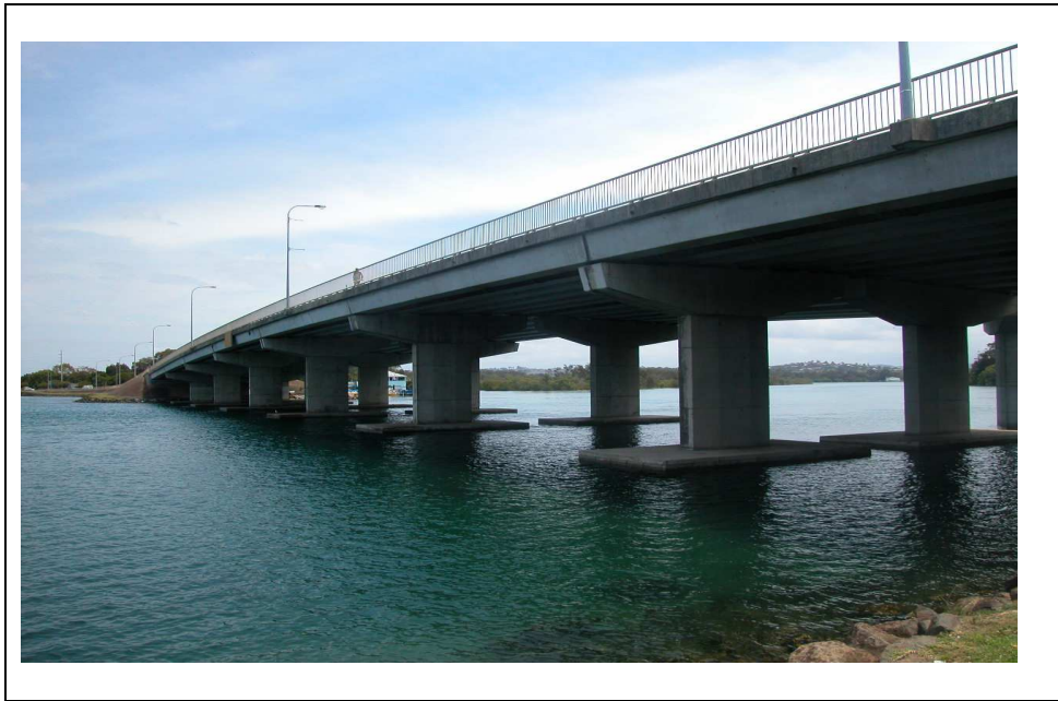
Figure 8 – Boyd's Bay Bridge. Located on the Tweed River, Tweed Heads
