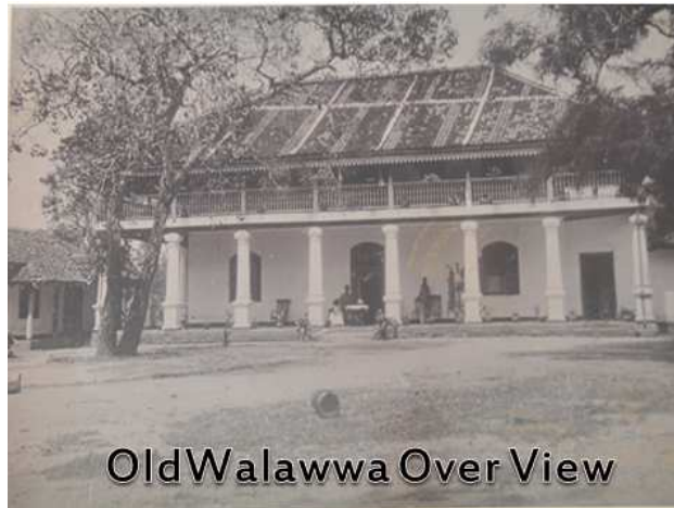
Figure 1: The bungalow prior to restoration
