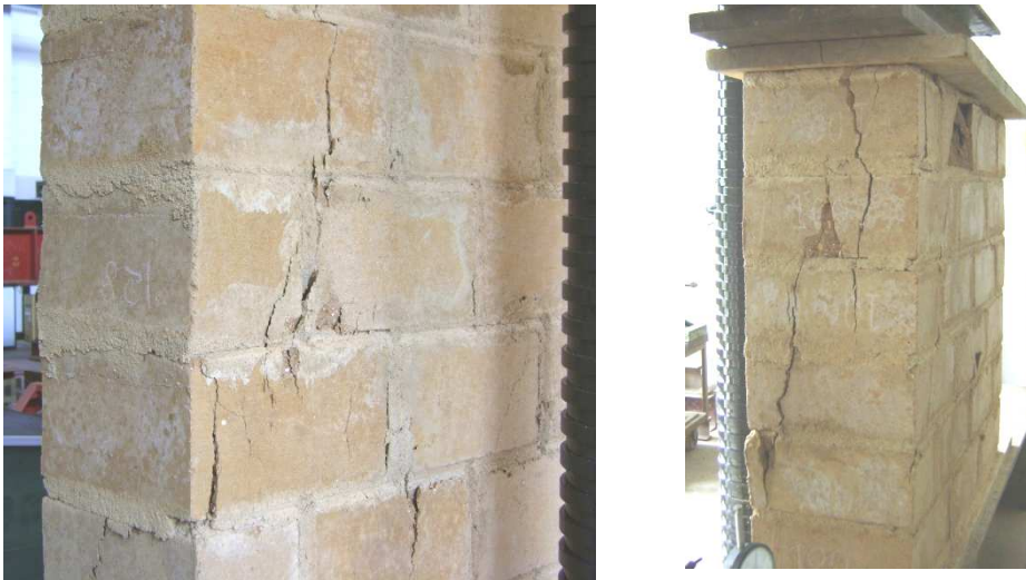
Figure 5 - Test panels after ultimate failure
