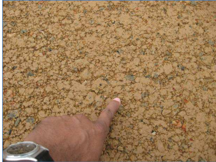
Figure 4: The light colour road surface without significant cracks
