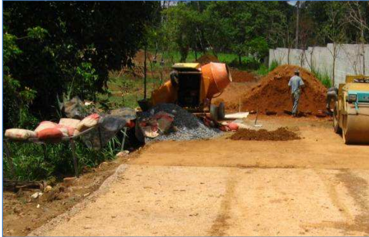
Figure 2: Cement and soil mixed with desired ratio
