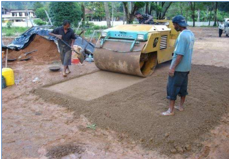
Figure 3: Five Ton roller was used for compaction
