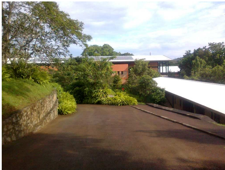
Figure 7: One of the main access road
