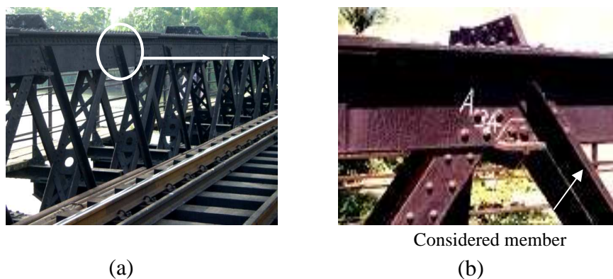
Figure 3: Views of (a) the bridge; (b) considered member
