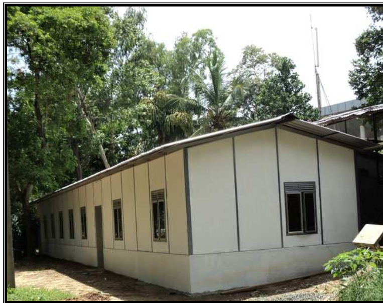
Figure 1: A building constructed with “Dura” panels and steel channels to be used as a site office
