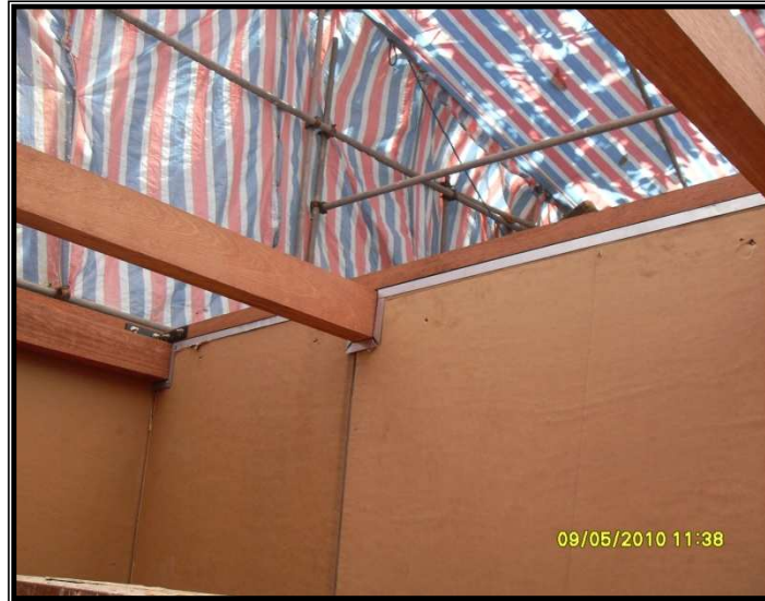
Figure 6: The beam arrangement for supporting floor slabs made by Dura panels
