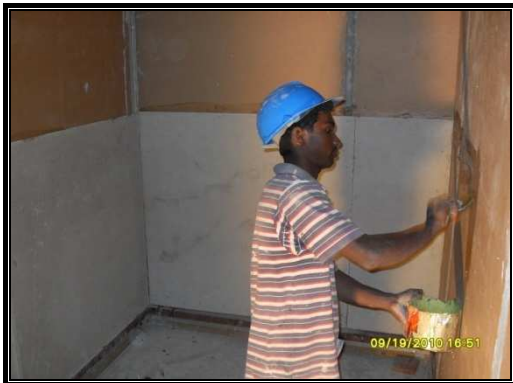
Figure 11: Additional water-proofing provided with fiber cement boards
