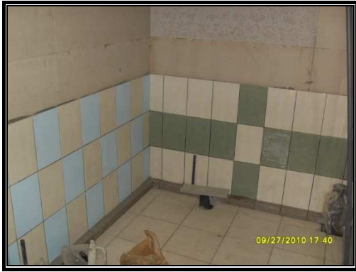
Figure 9: Bathrooms provided with a tiles to ensure proper water proofing
