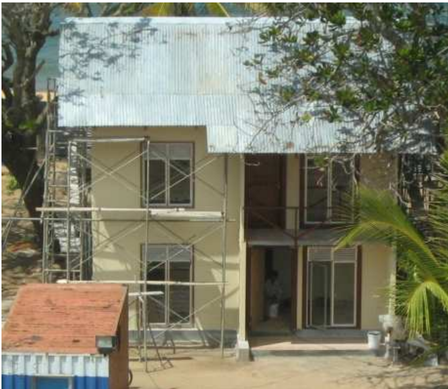
Figure 8: The two storey house under construction
