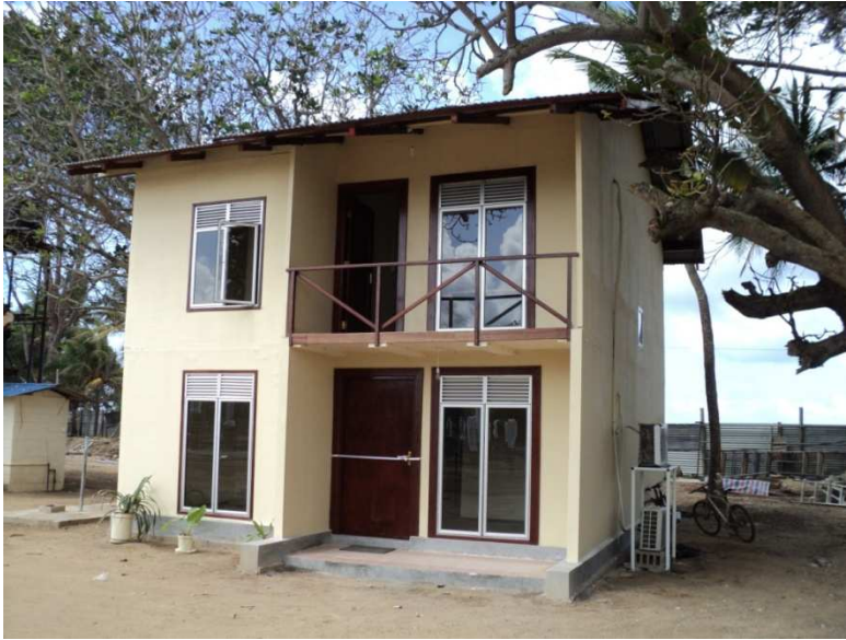
Figure 7: The two storey house that has been constructed with Dura panels being used for ground and upper floor walls, floor slabs and the insulation in roof
