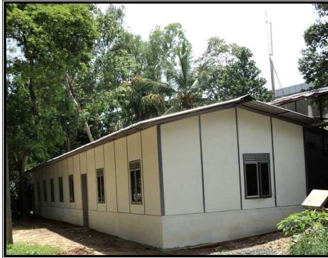
Figure 3: Panels that have been fixed using galvanized steel channels in a site office
