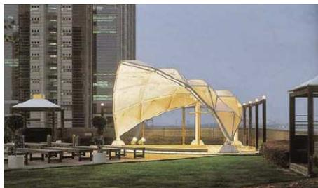
**Fig.12:** This fabric membrane structure at the Hyatt Regency in Osaka uses a photocatalytic clear coat based on  $\text{TiO}_2$ , which creates antibacterial effect. (Ashby *et al.*, 2009)
