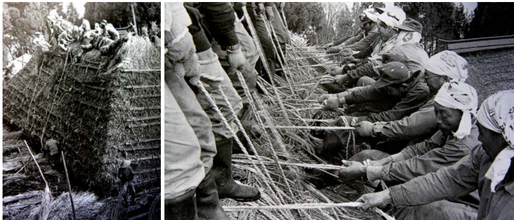
Figure 4: Picture of thatched roof Fushin,worked community peoples cooperated. (Sudou, 2004)
