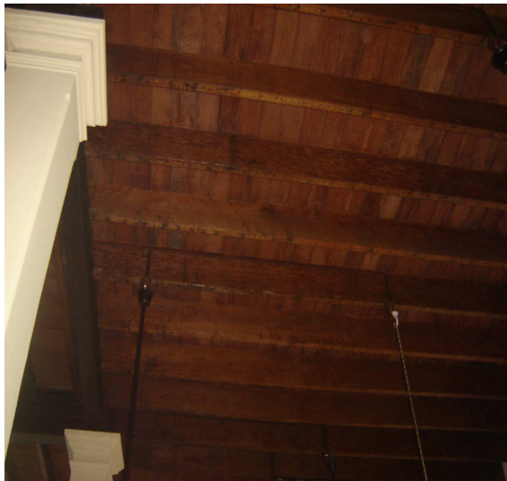
Fig 3.1 The timber floor of Dutch Burger Union, Colombo
