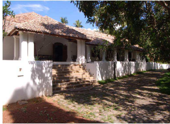
Fig 5.4 – Bungalow at Kakenadura, Matara after renovation
