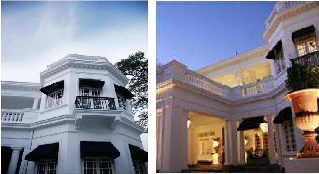
Fig 5.6 – Building at No. 65, Rosmead Place after renovations
