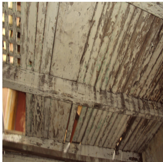
Fig 2.2 – The timber floor of an Old building in Galle Fort
