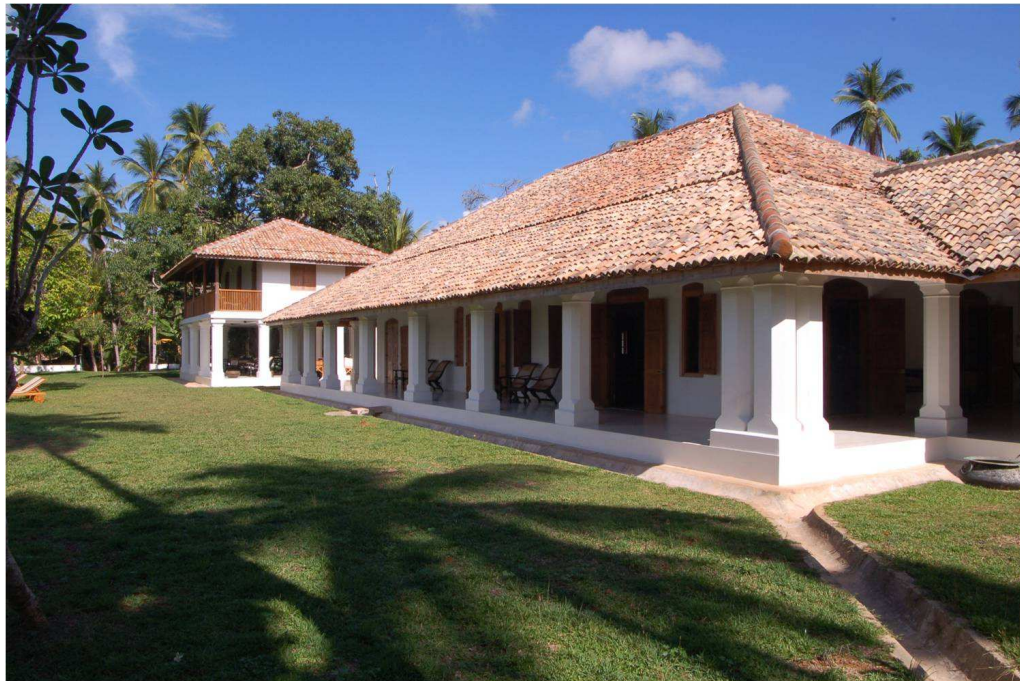
Fig 5.5 – Bungalow at Kakenadura, Matara after renovation
