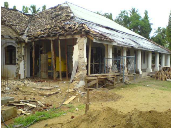
Fig 5.3 – Bungalow at Kakenadura, Matara before renovation
