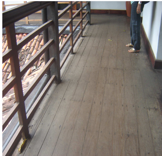
Fig 3.2 Timber used for external corridor of Dutch Burger Union, Colombo
