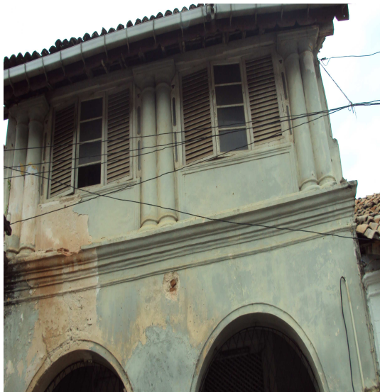
Fig 2.1 – An old building in Galle Fort planned for renovation
