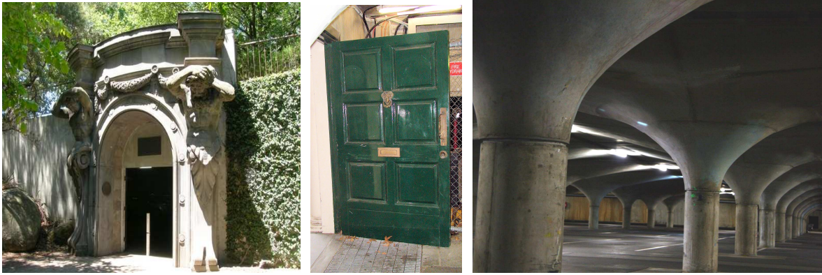
Figure 2: The two entrances (both examples of reuse options) and the Underground Car-park at The University of Melbourne
