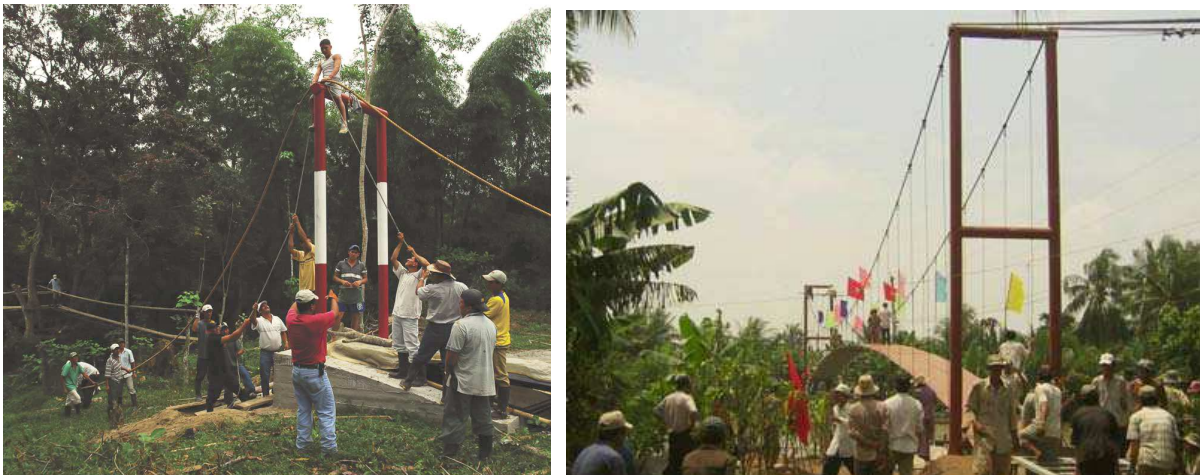
Figure 4: Rüttimann's Suspension Bridges– under construction (Ecuador), completed (Vietnam)
