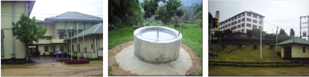
Figure 9: Hotel biogas plant and the Natural beauty after project
