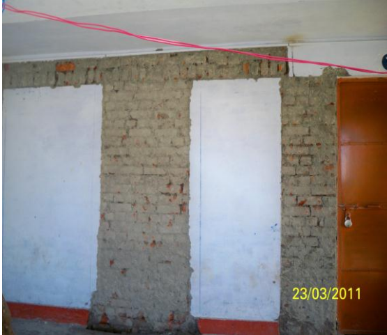
Fig.7 Racking of joint
