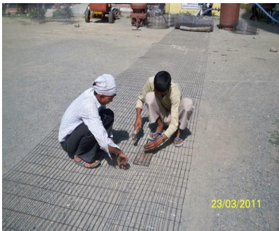
Fig.9 Preparing WWM as per Design
