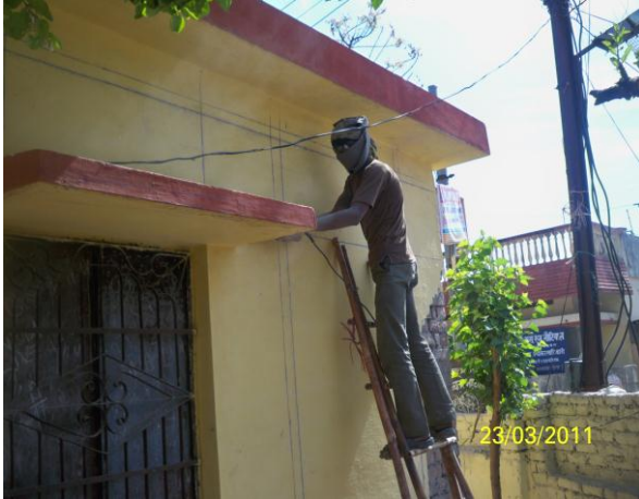
Fig. 5 Marking on Masonry Wall
