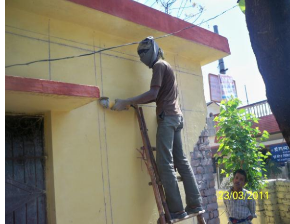
Fig. 6 Mechanical cutter used for cutting plaster
