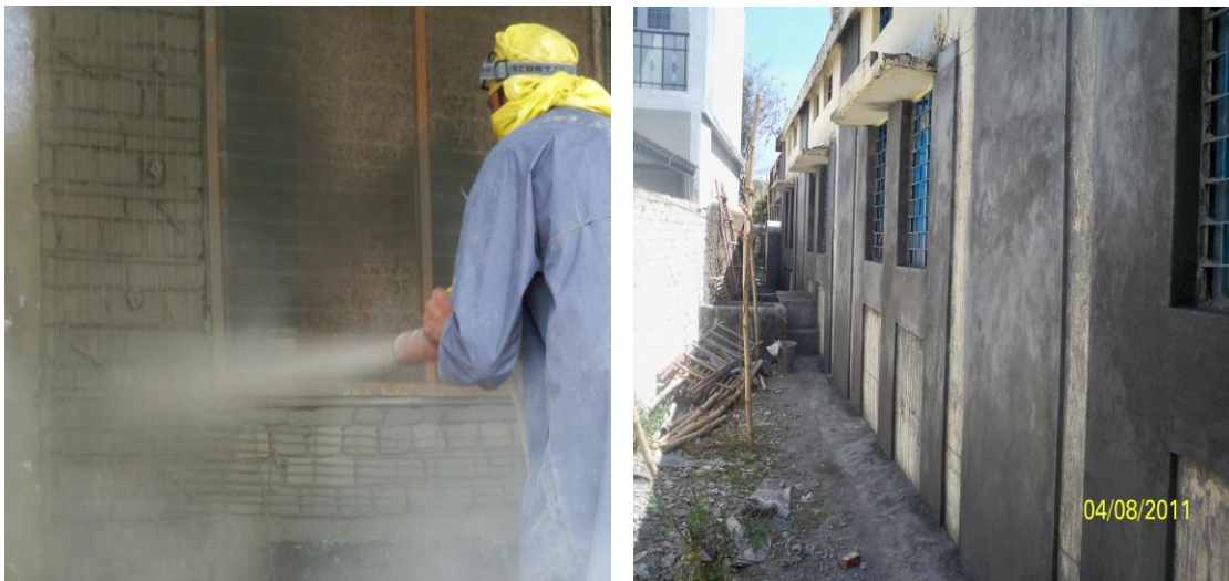
Fig.11 Gunitting operation and final view after second layer.
