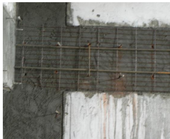
Fig.10 Fixing of WWM Mesh for Bandage
