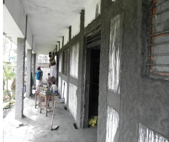
Fig.8 First Layer of micro concrete
