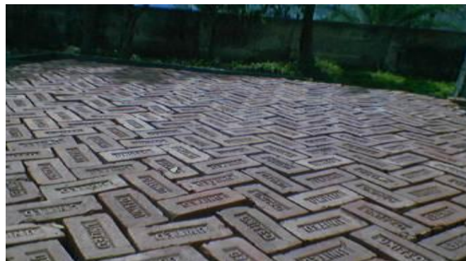
Figure 6: Photograph of Close view - showing the interspaces 12.7mm in bricks
