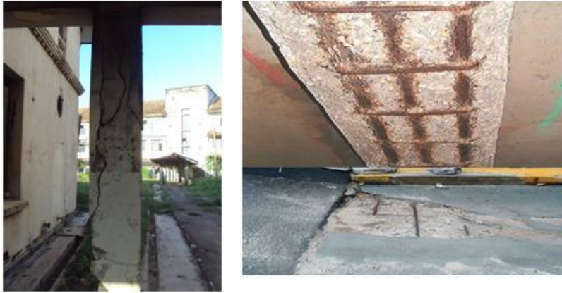
Figure 2: Deterioration Process of RC structures due to corrosion.
