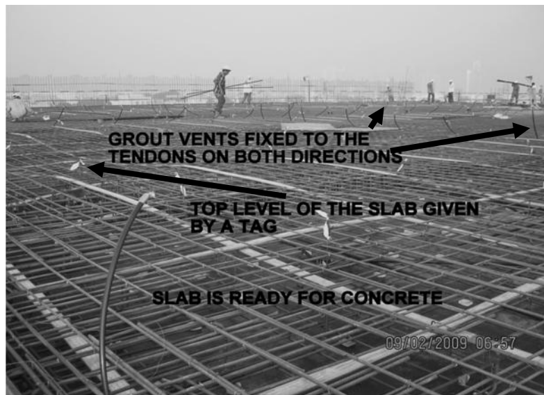
Figure 7: Fixing of Grout Vent
