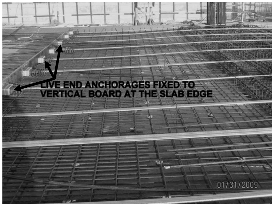
Figure 2: Practical usage of the Live End Anchorage at site
