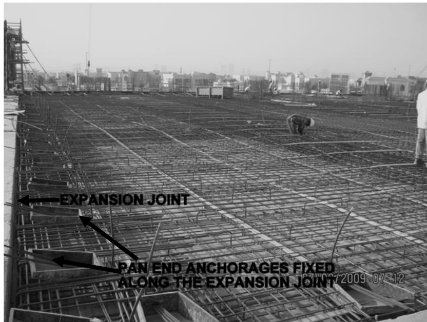
Figure 1: Practical usage of the Pan End Anchorage at site
