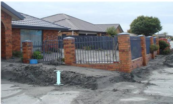
Figure 6 Houses that settled and have been inundated by ejected material in a major liquefaction zone
