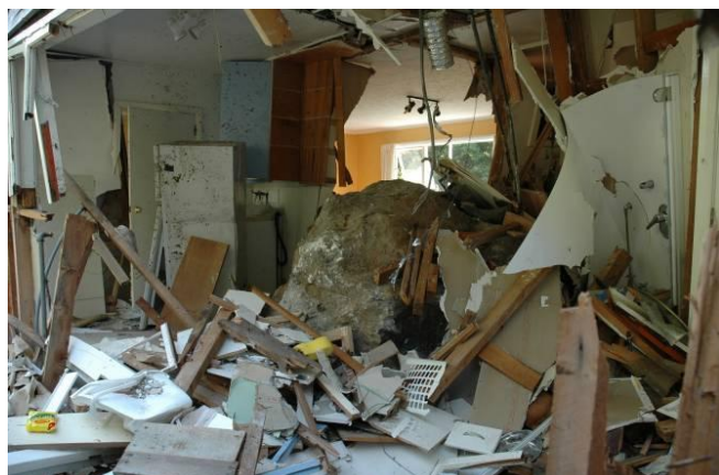
Figure 4. House damage in Heathcote due to rock fall (Carradine)
