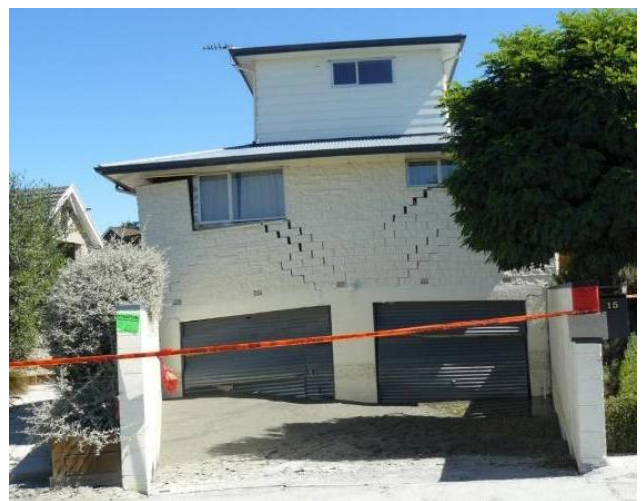
Figure 7 Masonry veneer damage due to lateral spreading and differential settlement (Buchanan) and due to differential settlement
