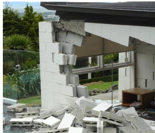
Figure 19 Left: Collapse of unreinforced masonry exterior wall (Carradine), and Right: Collapse of unreinforced masonry exterior wall (Morris)
