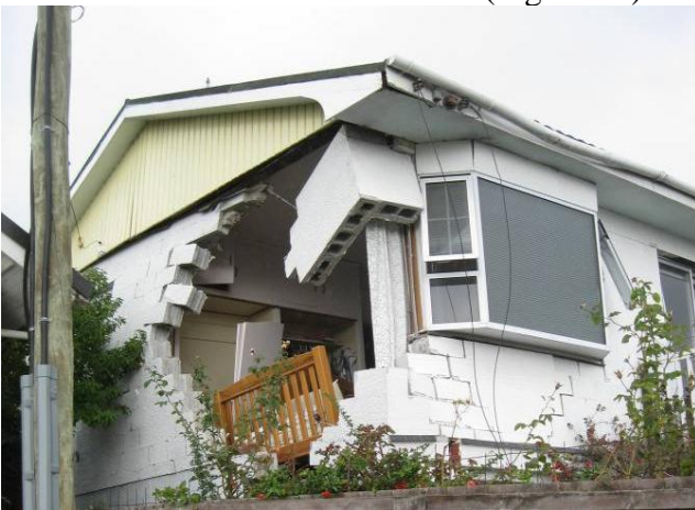
Figure 19 Left: Collapse of unreinforced masonry exterior wall (Carradine), and Right: Collapse of unreinforced masonry exterior wall (Morris)
