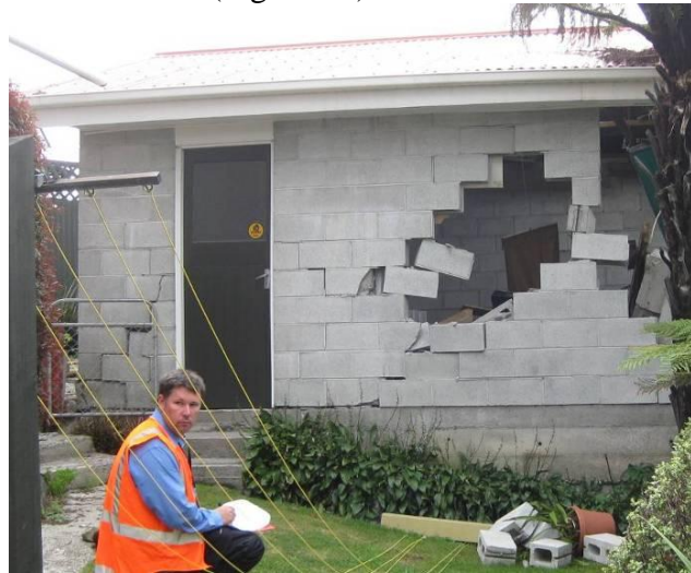
Figure 18 UngROUTED cells with reinforcing steel in place (Beattie)
