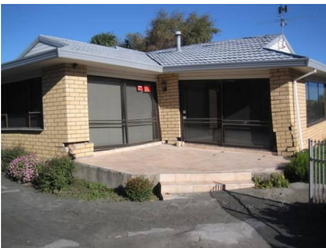
Figure 7 Masonry veneer damage due to lateral spreading and differential settlement (Buchanan) and due to differential settlement
