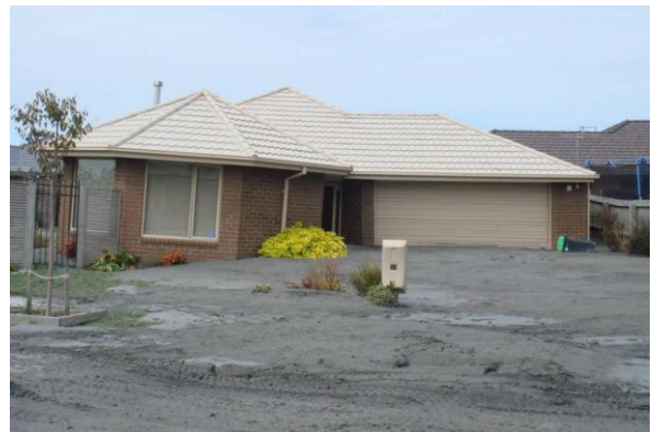
Figure 6 Houses that settled and have been inundated by ejected material in a major liquefaction zone
